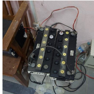
Figure 13 - Battery placement, Need cross ventilation.
