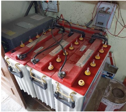
Figure 13 - Battery placement, Need cross ventilation.
