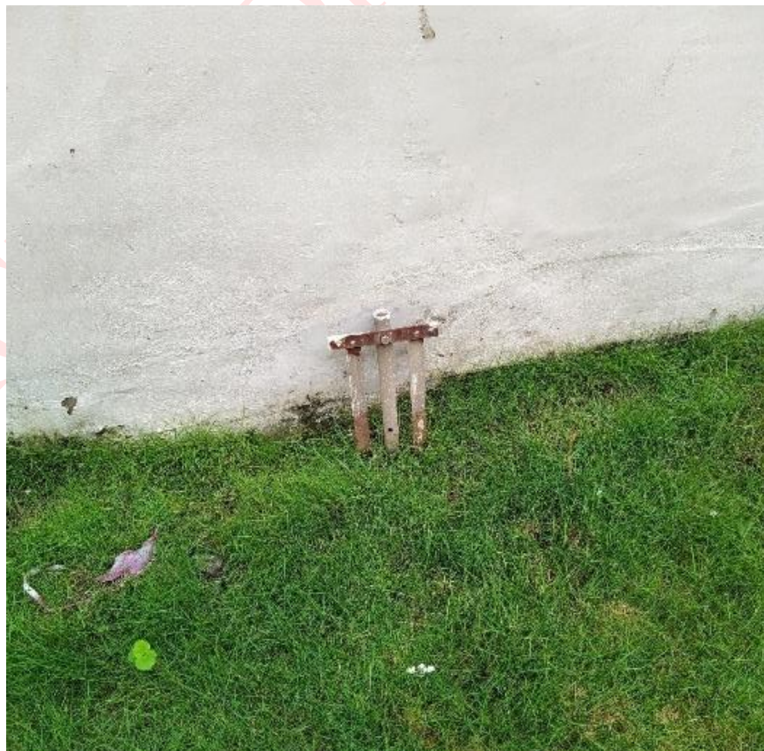
Figure 15 - Safety, electrical earthing compliance
